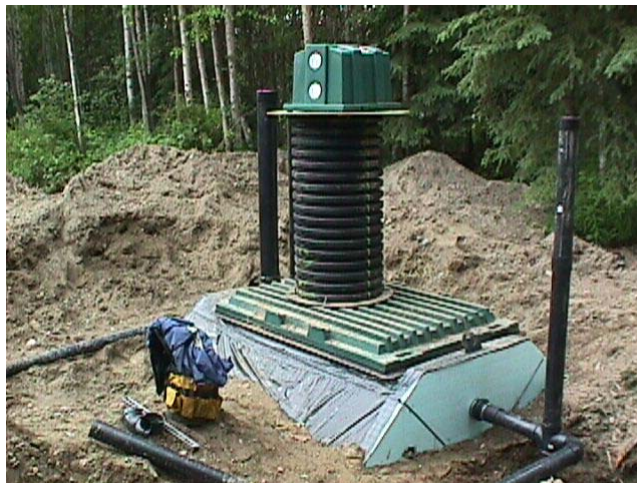
Photo shows a USTP300AT (aerobic treatment compartment only)
